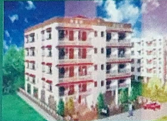
Panvasho Enclave Ashokpuri, Khajpura, Patna
